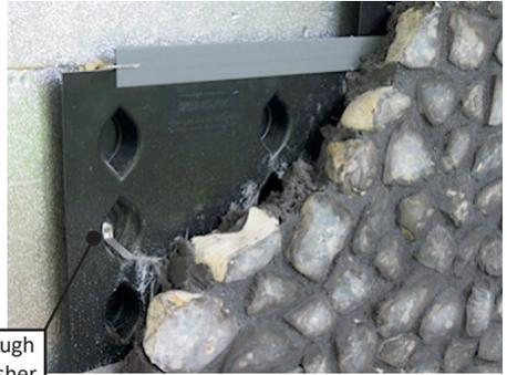
Additional tie, fixed through the pod using a seal -washer
