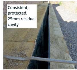
**SureCav25 is the only accepted way to build a 25mm residual cavity!**
